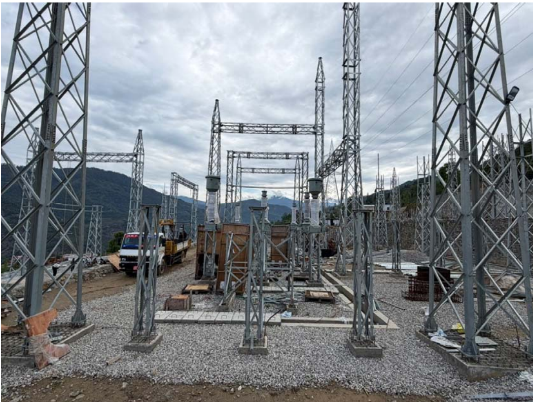
Installation of the Sub station EM equipment at LILO by EM team
