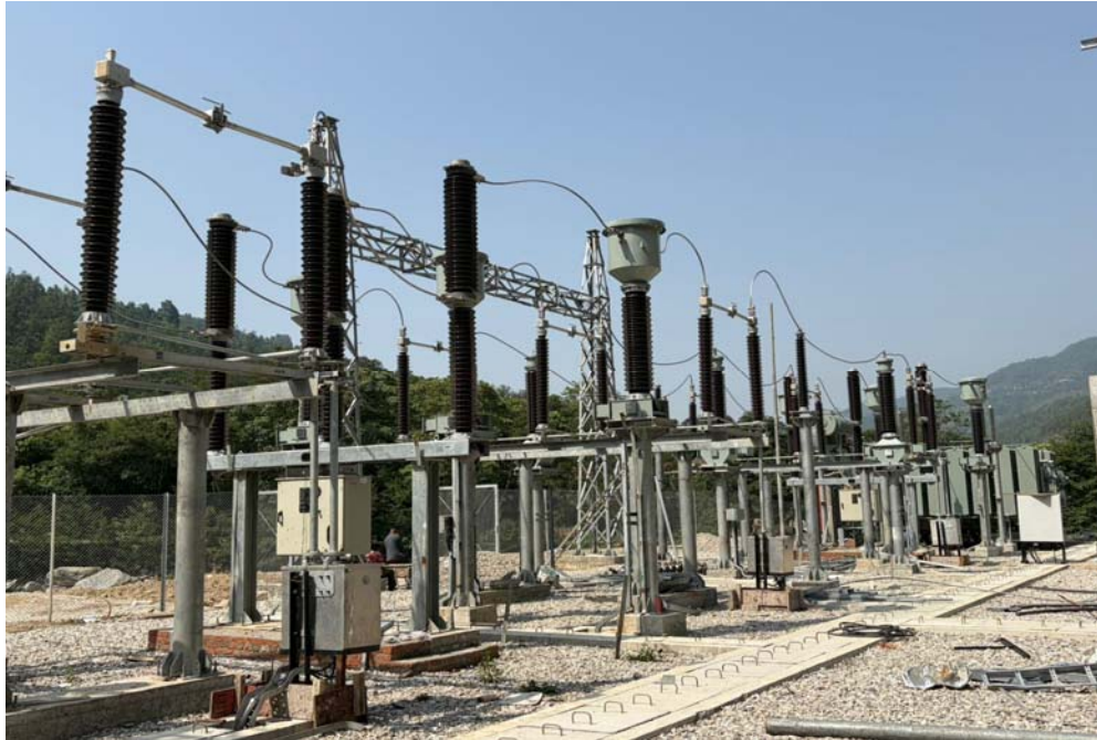
Outdoor 132Kv equipment connection works
