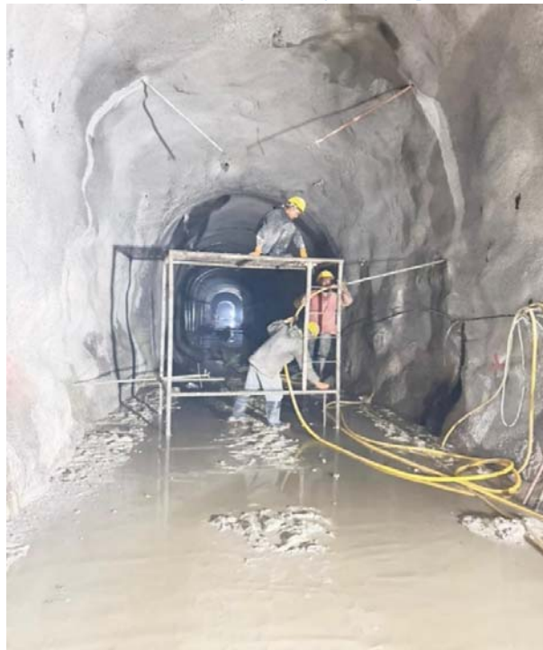
Consolidated grouting work at Face 2
