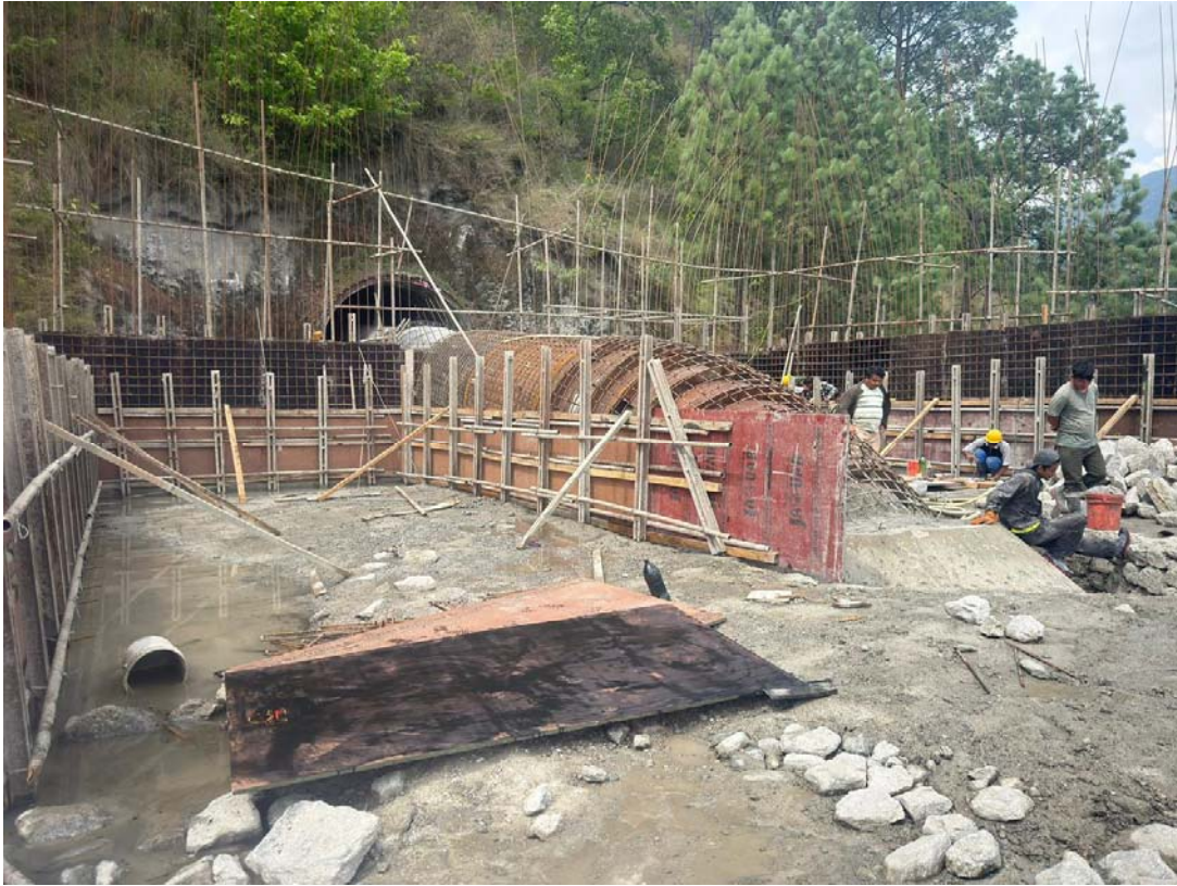
Anchor Block (AB06) Outside of the UPT
