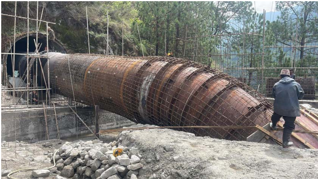
Completion of the Installation of Pipe by HM team at UPT
