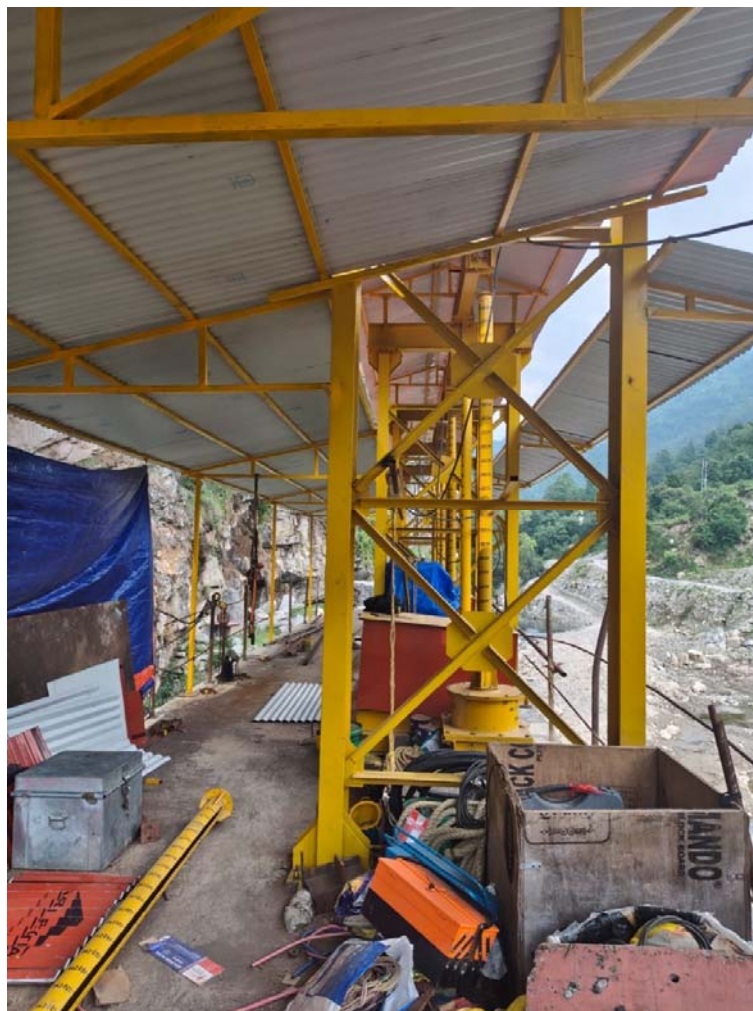
Super Structure work at the Headworks area
