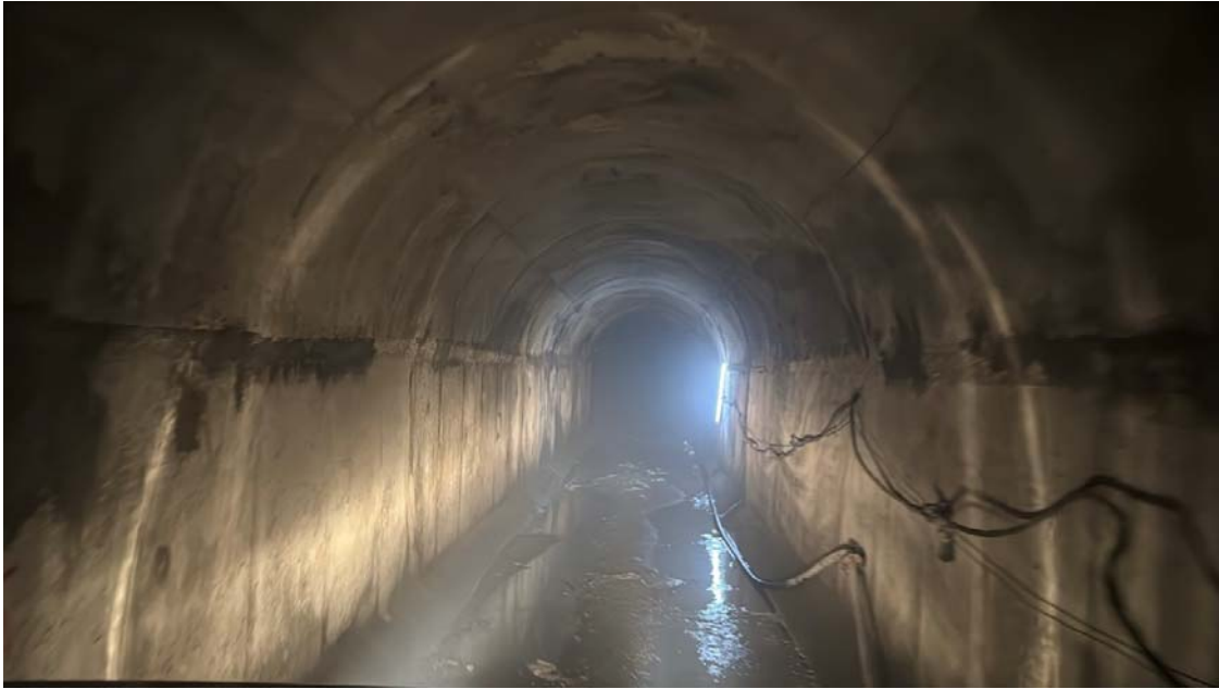
Face 1 Concrete lining work.
