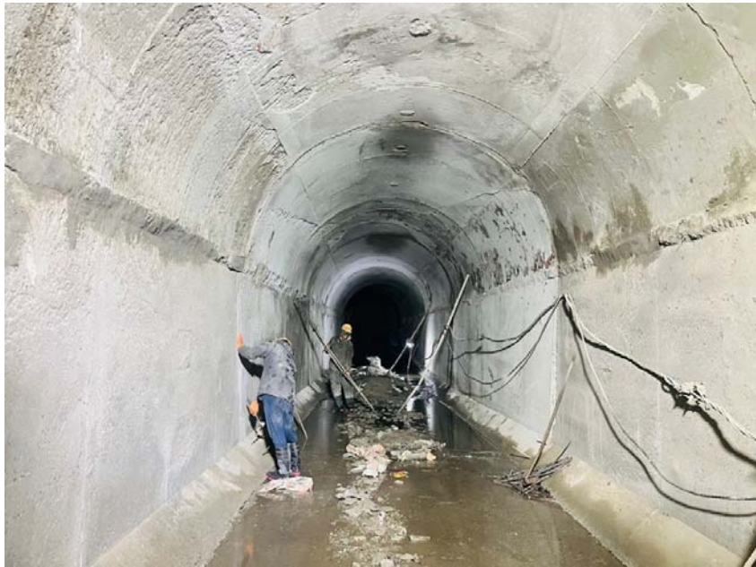
Face 2: Full lining work in face 2 completed
