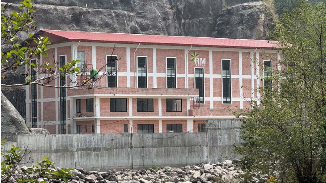
Power House of K2HEP
