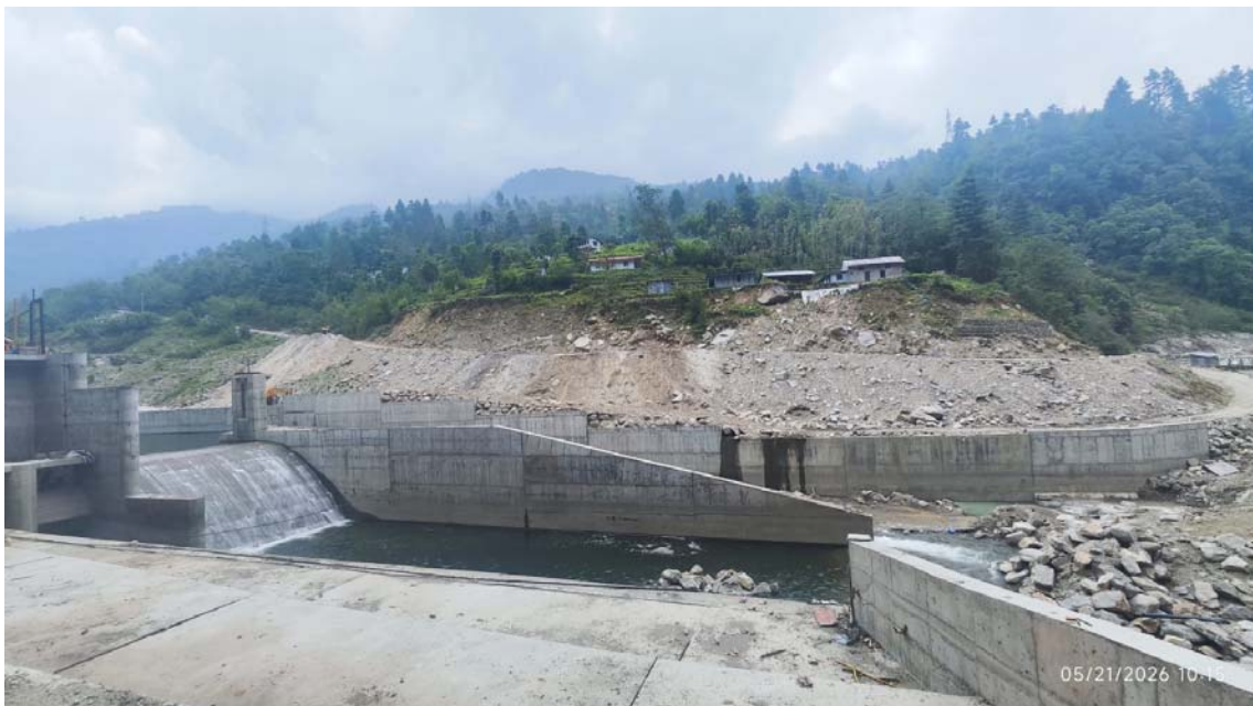
Left bank Back fill works continuous
