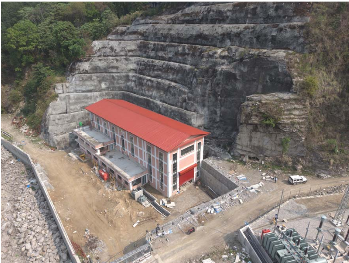
Figure: Overall View of Powerhouse
