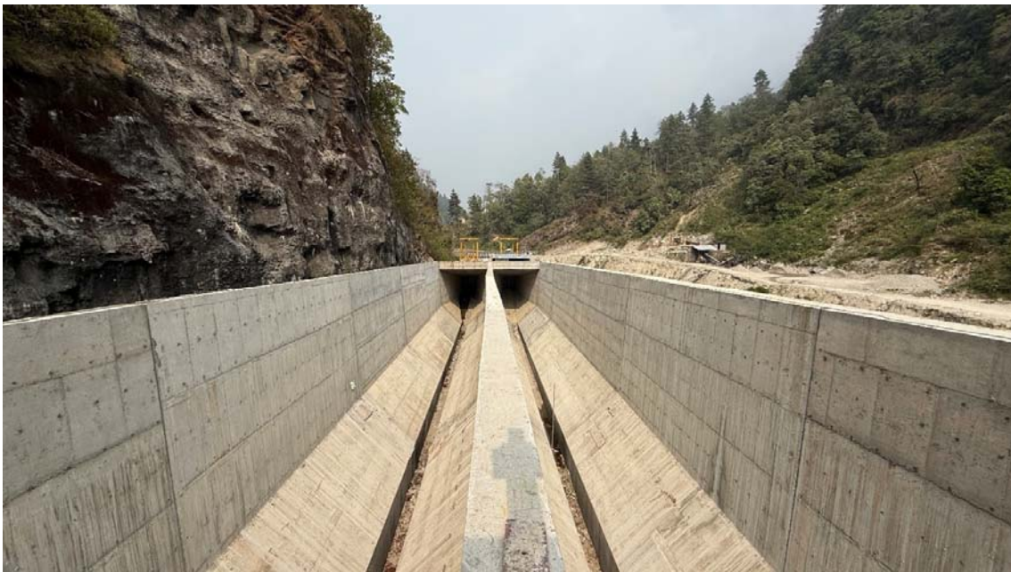
Overall, View of the Settling Basin
