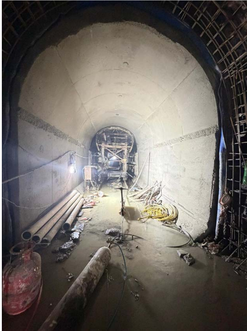
Full Concrete work in Face 3
