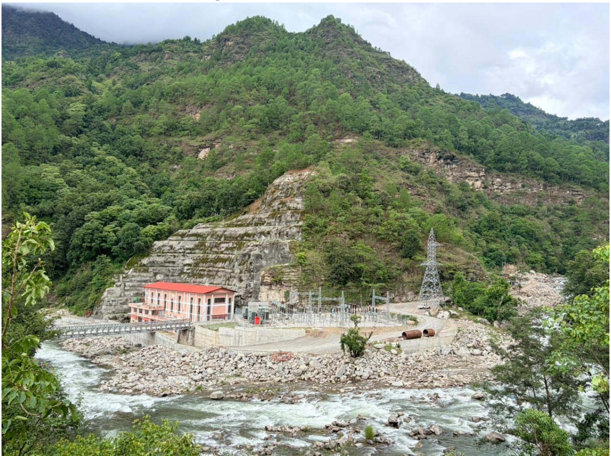
Overall Viwe of Powerhouse Area
