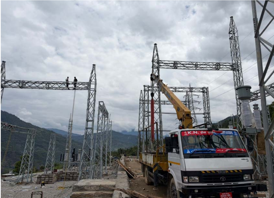
Beam erection processing at LILO
