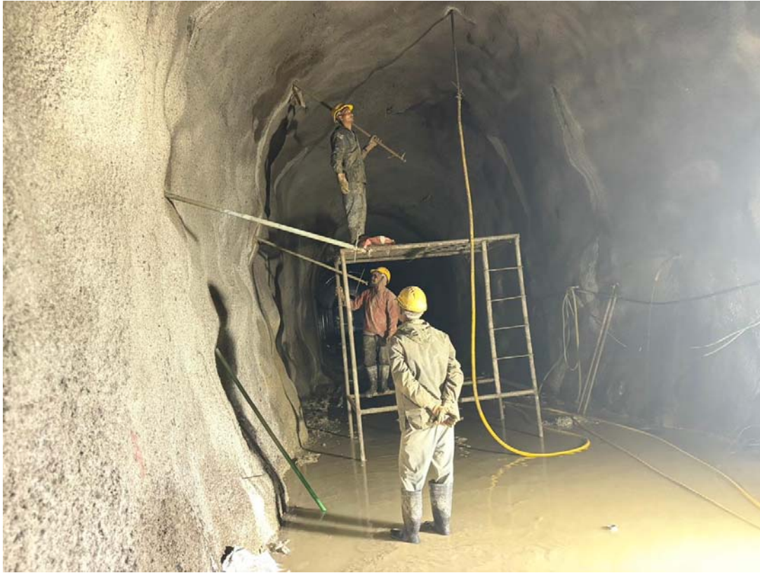
Grouting Work at Face 3
