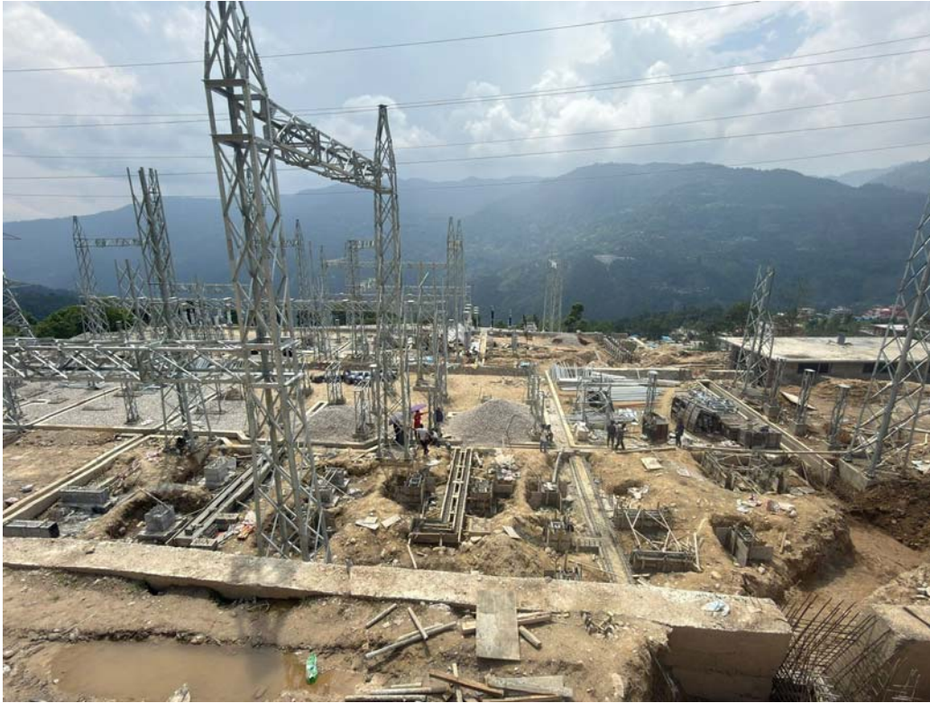
Various Structure foundation works
