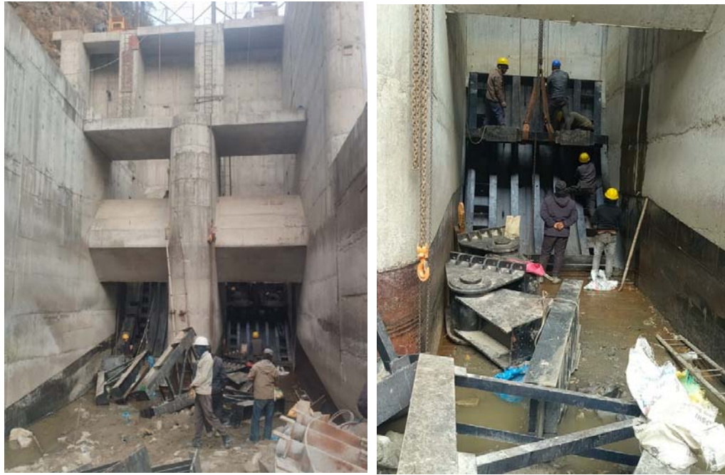
Radial Gate Installation work by HM team
