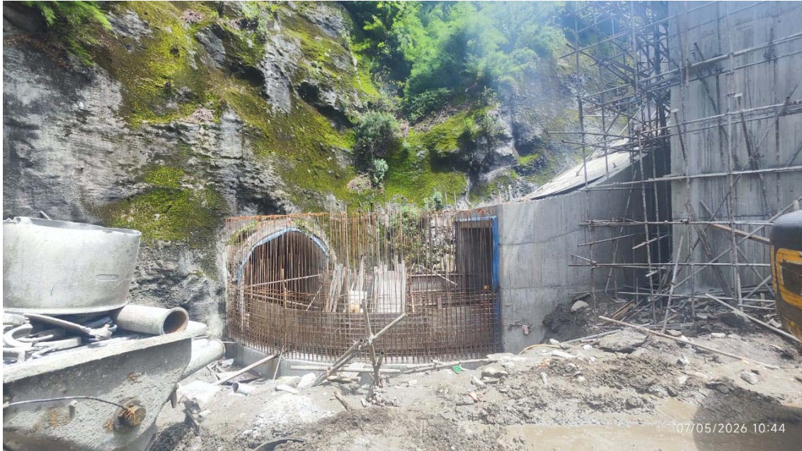
Transition part between head pond outlet and inlet
