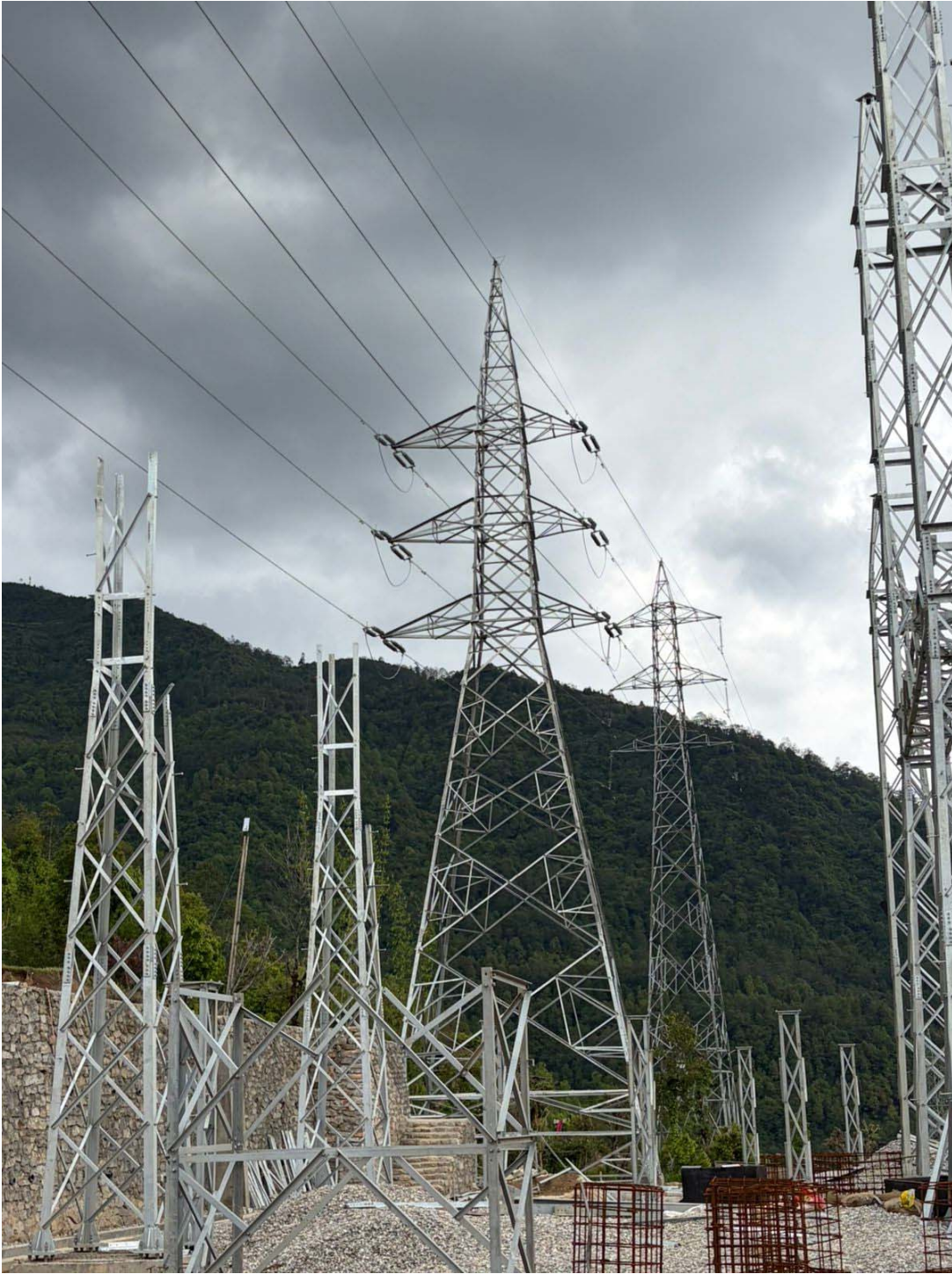
(Outgoing Tower) Completion of the erection of Dead End Towers
