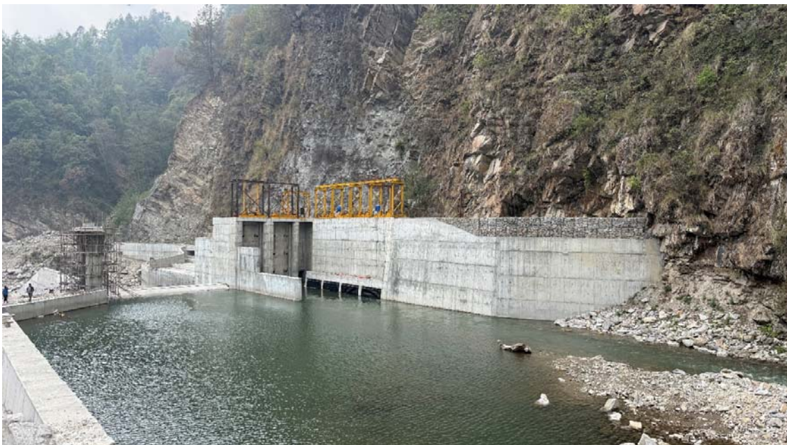
Overall, View of the Headworks Area
