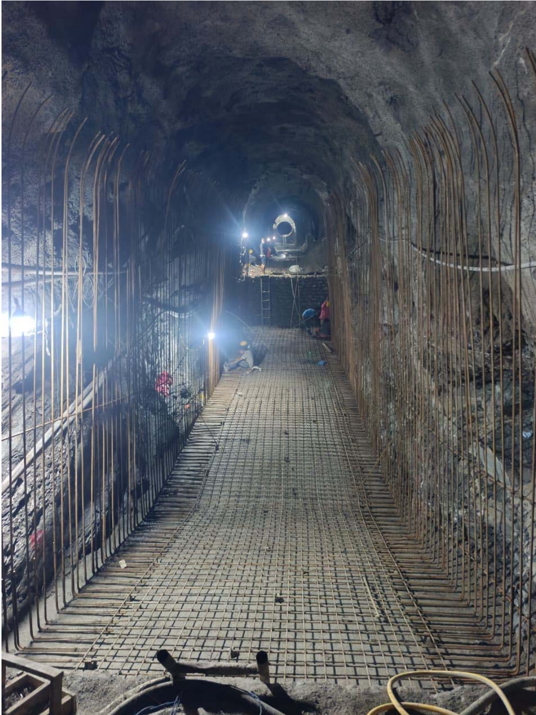
Rock Trap Rebar work
