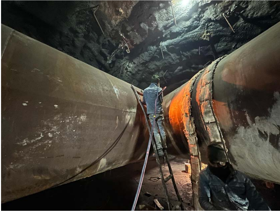
Pipe Installation work at T Junction
