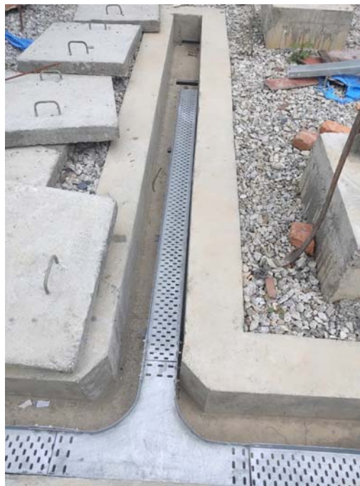
Cable tray installation and above ground earthing work
