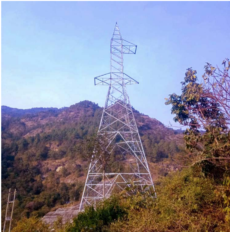
AP2 Tower at Powerhouse Switchyards
